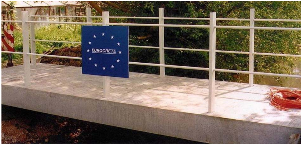
Figure 1-1: The first concrete footbridge in Europe with only FRP reinforcement (EUROCRETE project)
